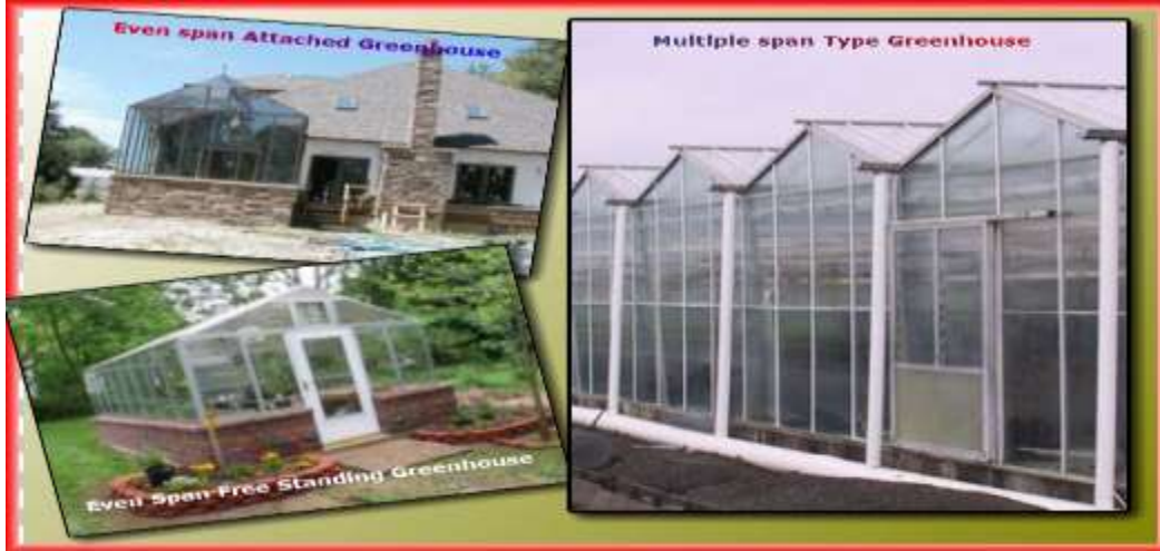
.Fig 1.3.2. Even Span Type Greenhouse
