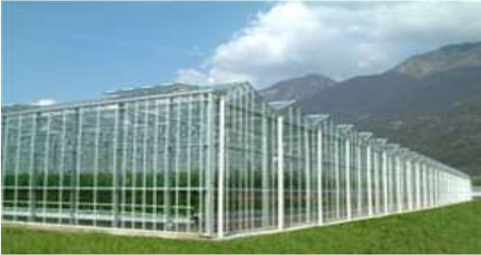
Fig. 1.3.4. Ridge and furrow type greenhouses
