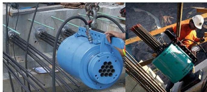
Figure 5: Details of a posttensioned beam
