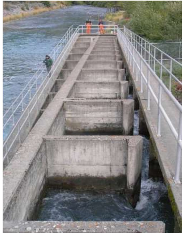
Fig (8-34) Vertical Slot Fish Ladder
