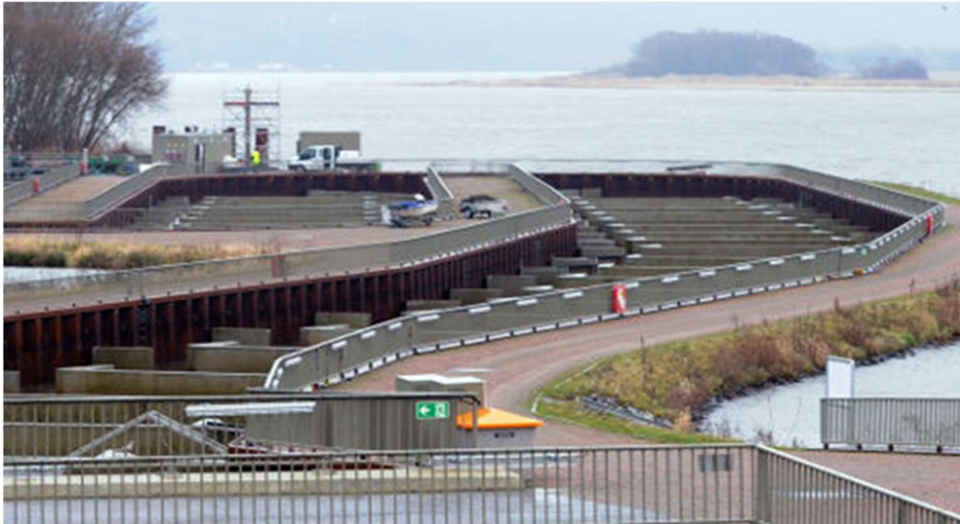
Fig (8-50) biggest fish ladder in the Elbe River near Hamburg
