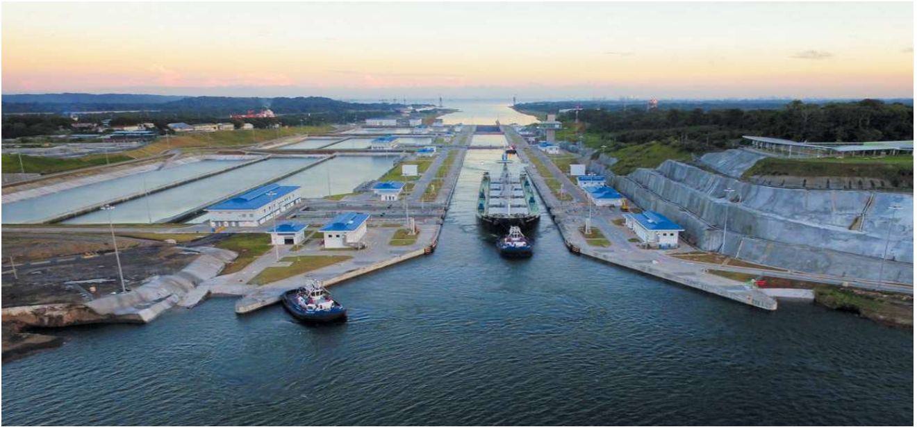
Fig (8-2) Panama Canal navigation
