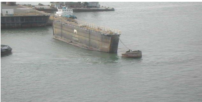
Fig (6.6) Graving Dry Dock Gate
