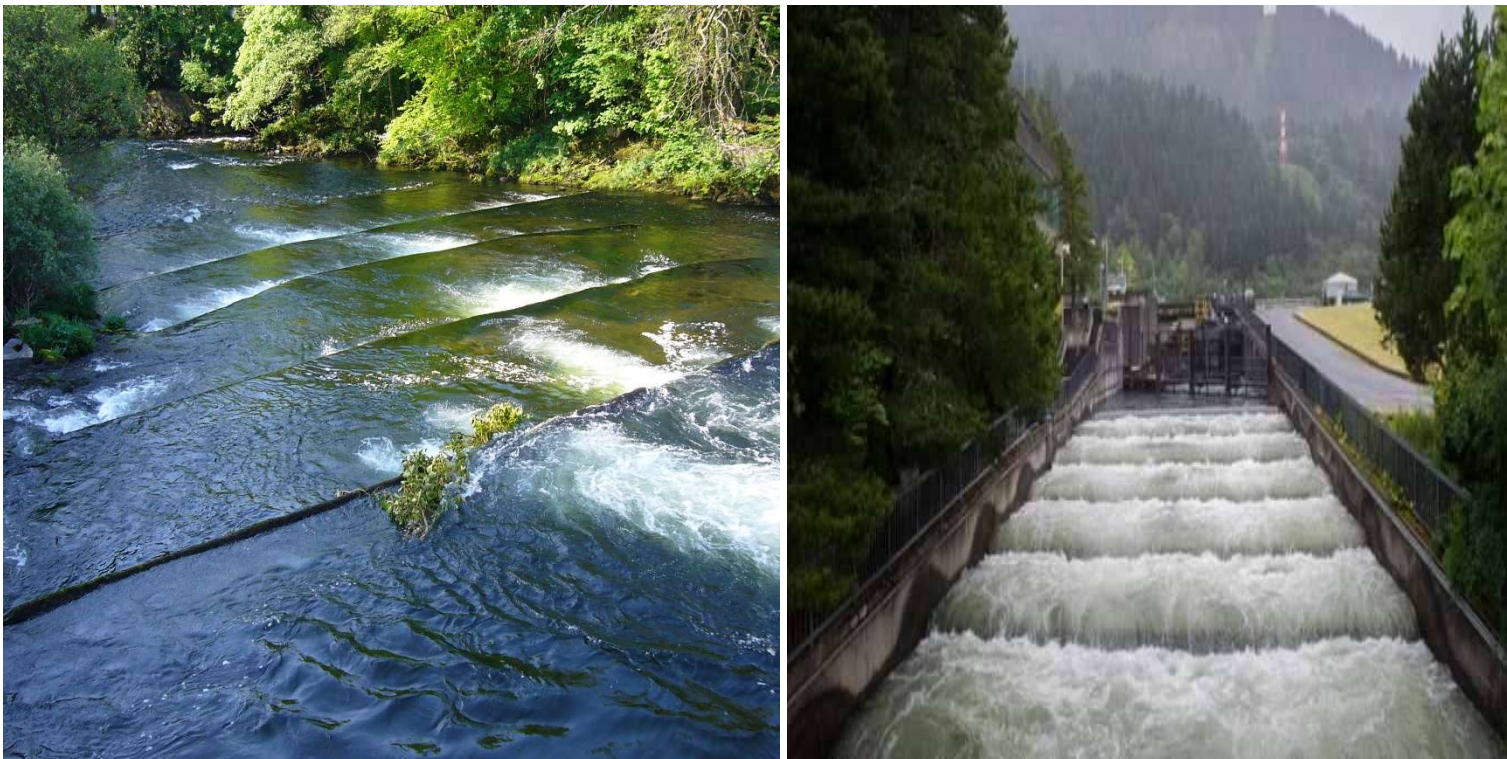
Figs (8-32) Pool and Weir type Fish Ladder
