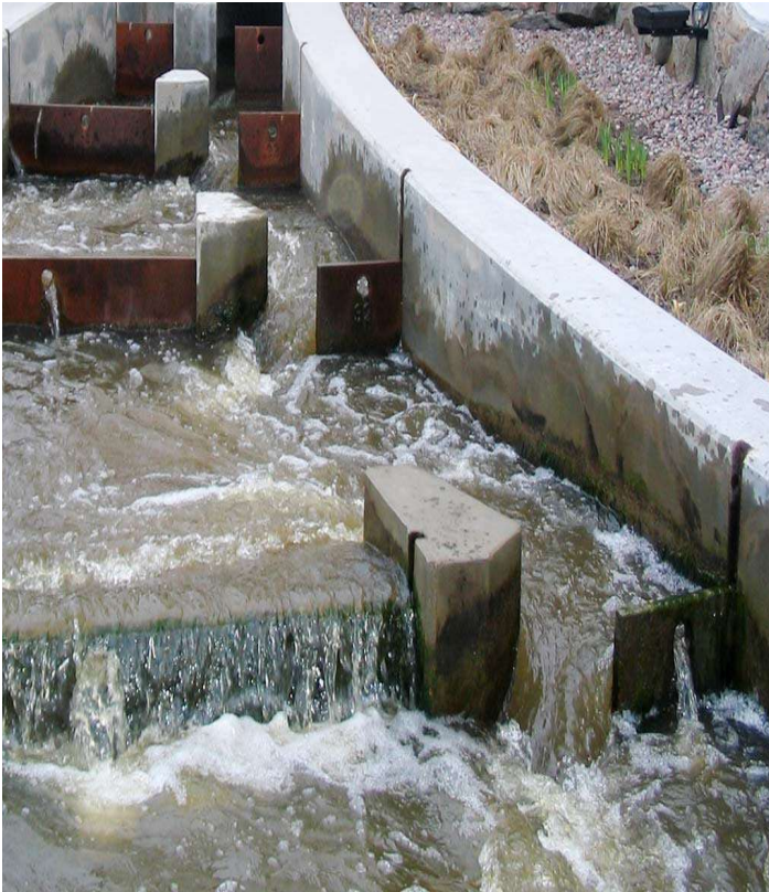
Fig (8-34) Vertical Slot Fish Ladder
