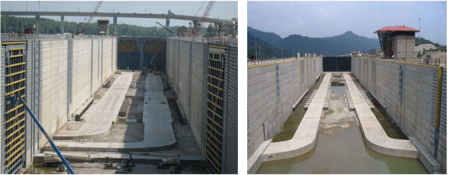
Fig (8-22) longitudinal culvert system
