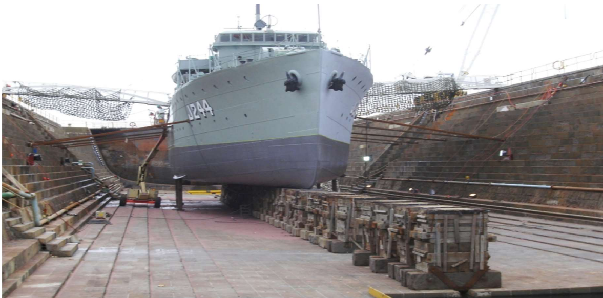
Fig (6.4) gravity dry dock
