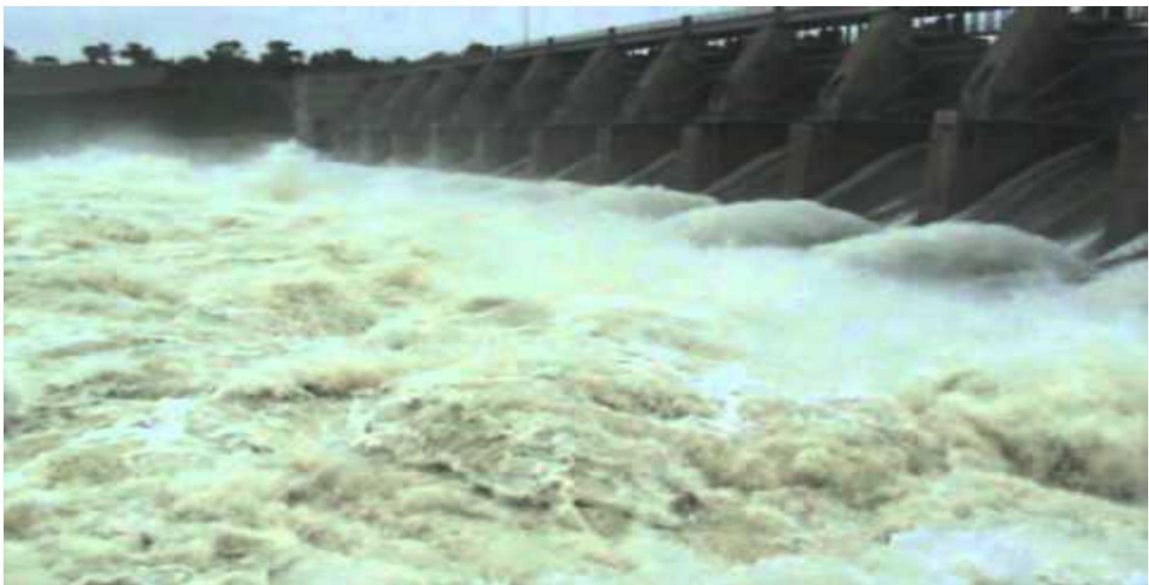
Fig.4.1 Hydraulic Jump
