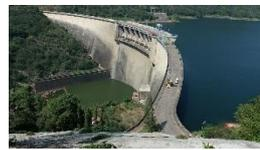
In constant radius arch dam, the upstream face of the dam has a constant radius making it a linear shape face throughout the height of the dam. But the inner curves their radius reduces as we move down from top elevation to bottom and thus in cross-section it makes a shape of a triangle.
