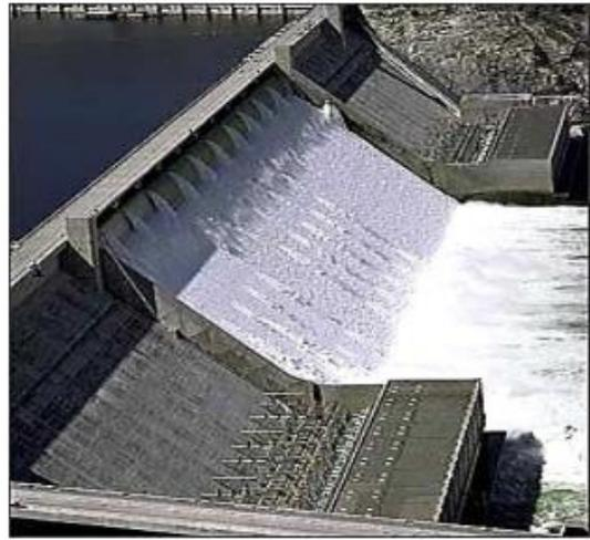
Concrete Gravity Dam ( over flow)
