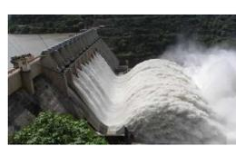
An outlet work may also act as a flood control regulator for releasing water stored temporarily in the space reserved for flood control. The outlets may also be used to empty the reservoir to make needed repairs or to maintain the upstream face of the dam or other structures.
