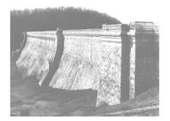
Masonry Gravity Dam (non-over flow)
