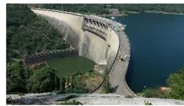
required thickness is proportional to its radius. Thickness relation in terms of intrados,  $r_i$  and mean radius  $r_c$ , can be derived as follows :
