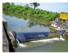
river bed. Generally, gravity drainage system is used for emptied of the rubber bag. So, it does not create obstruction for the passing of water in rainy season and also passage of boat freely through the River.
