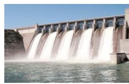
3. **Provision of sluices:** An adequate number of sluices should be provided at different levels in the dam to discharge sediment-laden water to the downstream.
