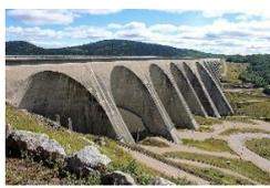
The sliding force is the horizontal component of hydrostatic force and the resisting forces are the vertical component of hydrostatic force and the concrete weight of dam.
