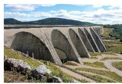
This type of dam can be preferred for larger heights about more than 50 meters. As compared to deck slab type buttress dams, multiple arch buttress dams are more flexible and stable.
