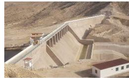
If ( $P_{max}$ ) exceeds the allowable compressive stress of dam material. (Generally taken as 3000 kN/m<sup>2</sup> for concrete; the dam may crush and fail by crushing.
