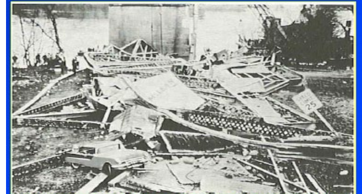
Collapse of Point Pleasant suspension bridge, West Virginia, 1967. May-Aug 2001
