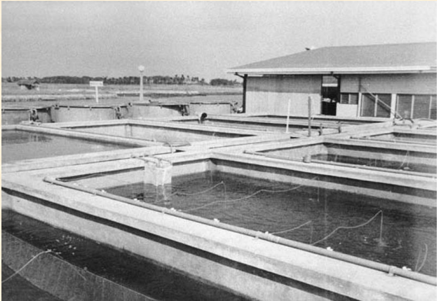
A hatchery system with spawning, nursery and rearing tanks.
