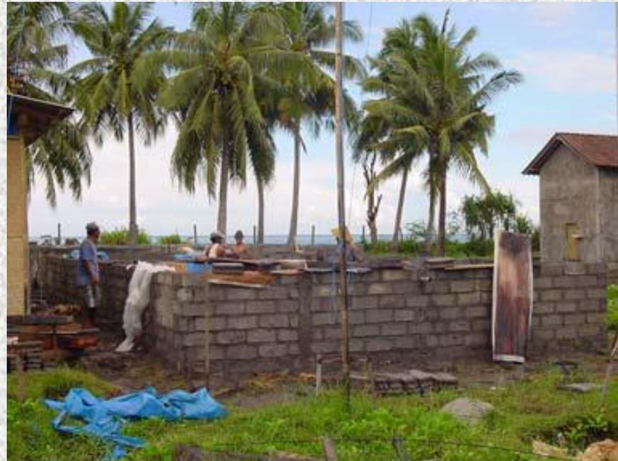
**Concrete blocks being used to construct rearing tanks for a small hatchery**
