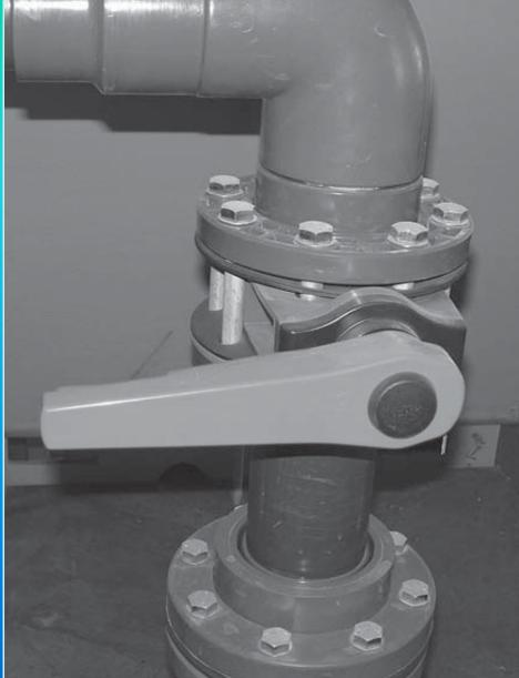
Ball valves are low cost solutions used in aquaculture. The disadvantage is that they are not very precise when regulating the water flow.
