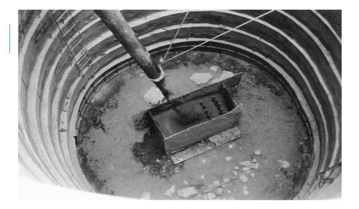
For concrete deposited in the formwork of walls, footings, beams, and shear walls, concrete **should be placed from the ends or corners toward the center**, **in horizontal layers not exceeding about 450mm in depth.**
