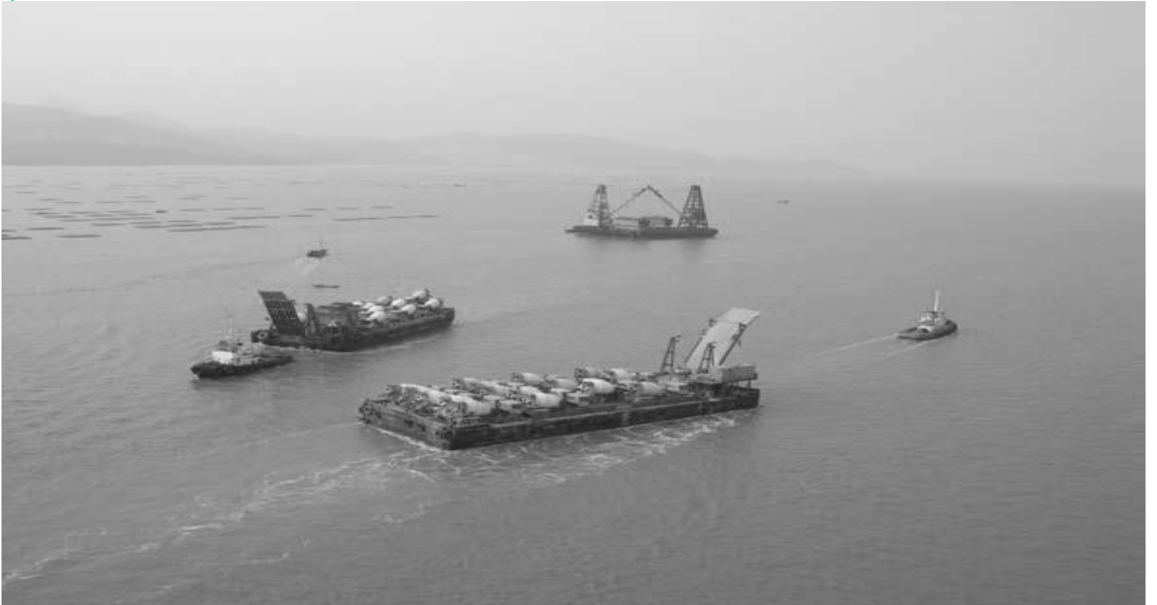
FIGURE 3-14 DELIVERY OF CONCRETE TO AN OCEAN CONSTRUCTION SITE USING A FERRY
