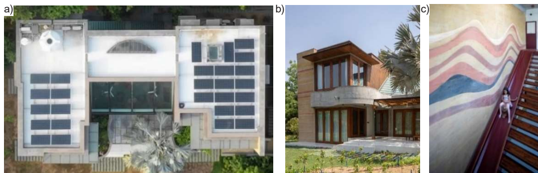
Fig. 25. Roof top solar panels (a), Large overhangs (b) and Rammed earth wall (c)
