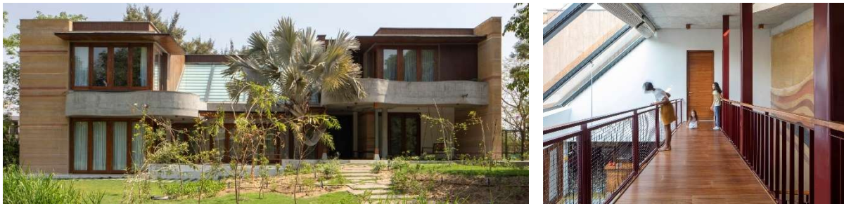
Fig. 23. External view of the house (Source: archdaily.com)
