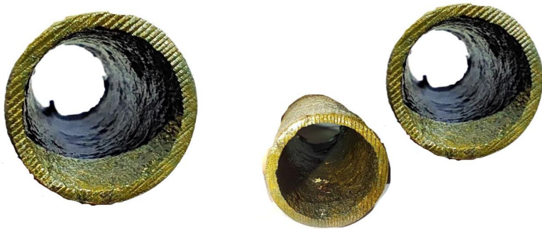
Figure 16. A sample of the heat exchanger pipe after treatment
