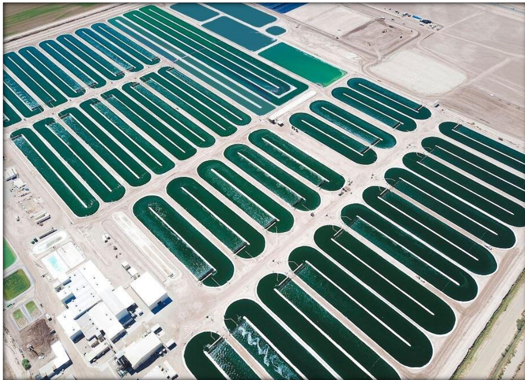
Fig. 1 Earthrise Farms Arthrospira production plant (Calipatria, CA, USA)
