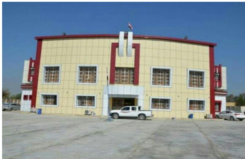
Figure 5: shows the facade of the building opposite the assembly area.
