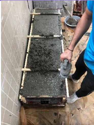
a. Compaction by rod vibration.
