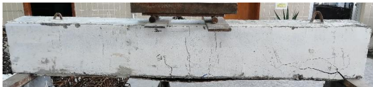
Fig. 14. RB0.7 Beam failure.
