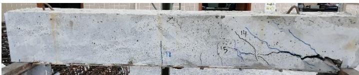
Fig. 12. SB5 Beam failure.
