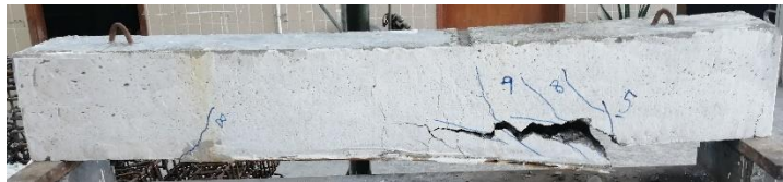
Fig. 9. SB2 Beam failure.
