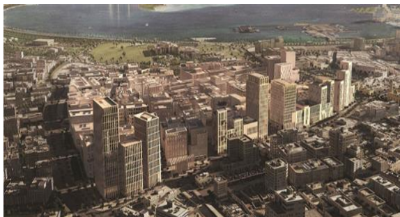
Figure 9. Aerial perspective showing the solidity and density of building blocks www.msheireb.com
