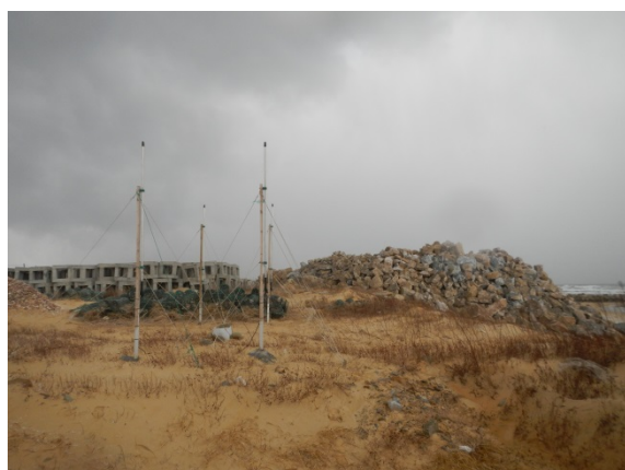
Figure 1. The cement blocks and stones on the coast waiting to be transported to the coastal waters for artificial reefs, the nearby is the HF radar transmit antennas.
