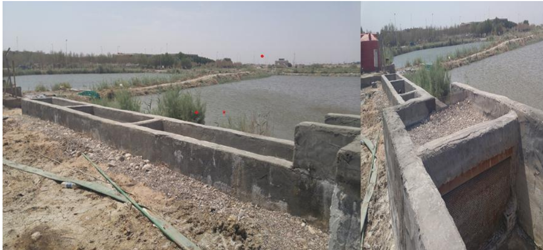
Pic. 9. The sand filter is connected to the storage pond in the shrimp farm.
