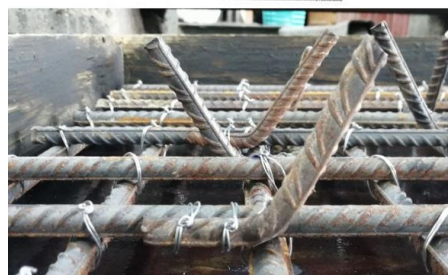
Figure 3. Y-type bar for shear reinforcement
