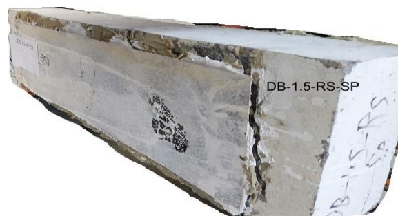
Figure (22): Failure mode for Rehabilitated Deep Beam with ( a/d=1.5 ) fail in shear - DB-1.5-RS-SP
