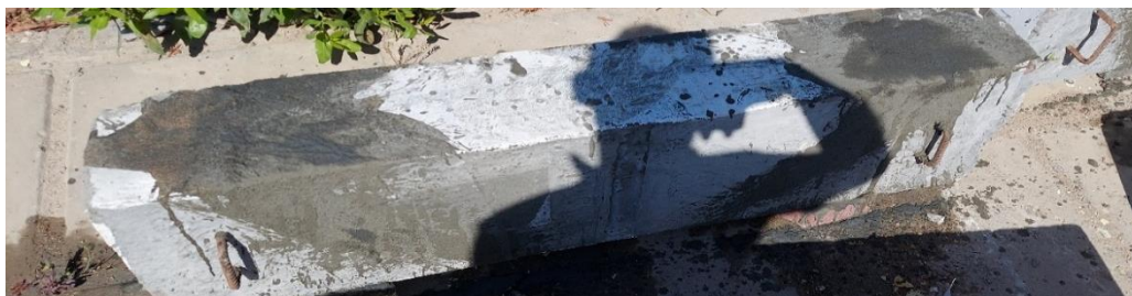
Fig (8). Repaired beams with cementitious grout
