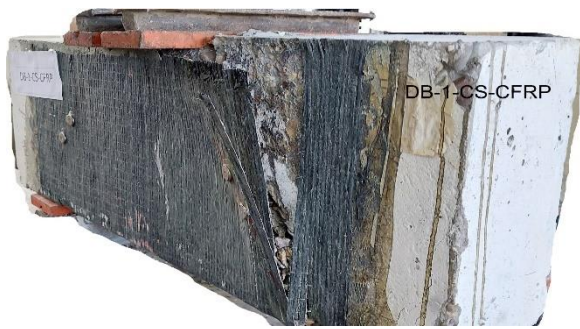
Figure (9): Failure mode for Rehabilitated Deep Beam with (a/d=1) failed in shear - DB-1-CS-CFRP
