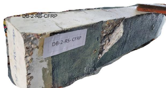
Figure (14): Failure mode for Rehabilitated Deep Beam with (a/d=2) failed in shear - DB-2-RS-CFRP
