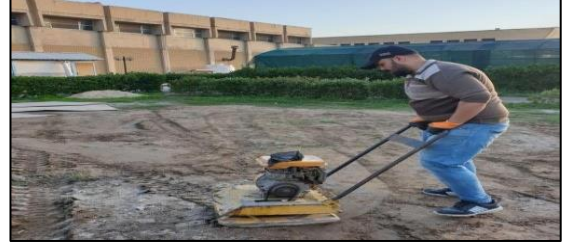
Fig.3. Ground leveling process
