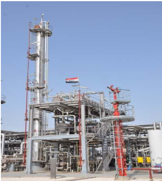
Fig. 1: UNIT 7501 in Basrah Refinery.
