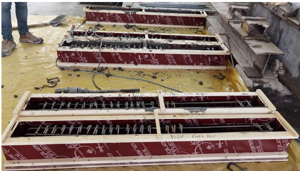
Fig. 4 Plywood forms, steel placing and concrete casting.
