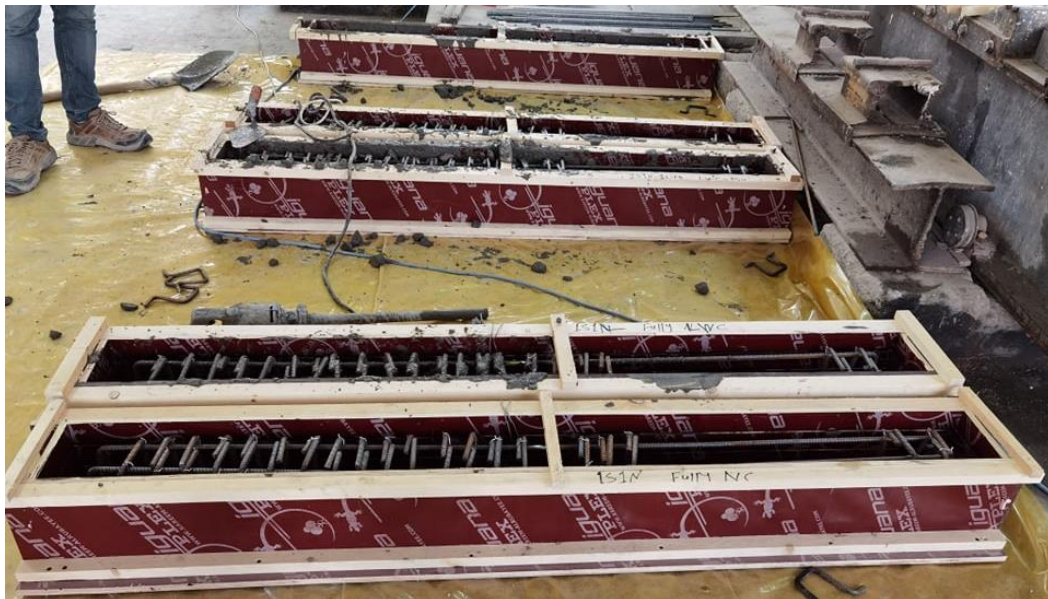
Fig. 4 Plywood forms, steel placing and concrete casting.
