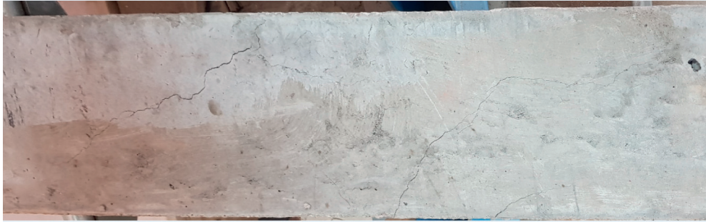
FIGURE 7: Crack pattern of steel fiber beam.
