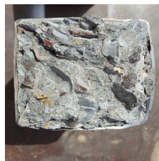
Figure 9: Concrete core after sever local buckling specimen SHS4
