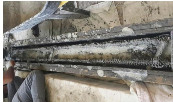
Figure 2: Beam casting
