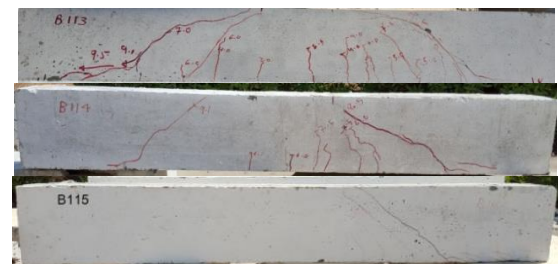
Figure 6: Crack pattern of group two ferrocement beams.
