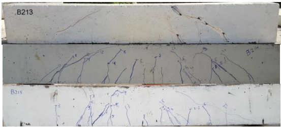
Figure 7: Crack pattern of group three ferrocement beams
