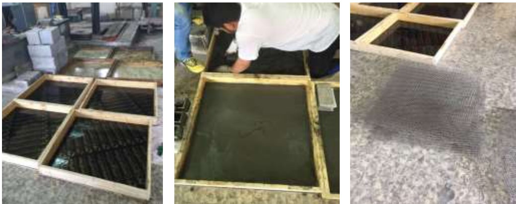
Fig 3: Placing the wire mesh and casting the slabs
