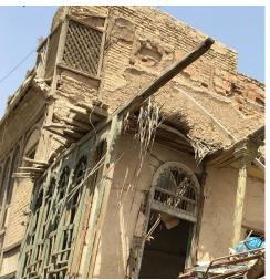
**Fig. 14:** A decayed roof showing the structural composition of the Jawi wooden ceiling of a Shanasheel building
