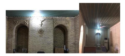
Fig. 15: A false ceiling covered with jawi wood in one of the Shanasheel buildings of the old city of Basra
