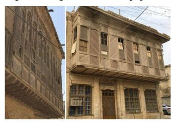
**Fig. 5:** Examples of Shanasheel base, one resting on wooden stands and the other on jack arch structure of iron and wood beams (newer) in the old city of Basra Source: Photos captured in the old city of Basra by the researcher on 1/9/2017.
