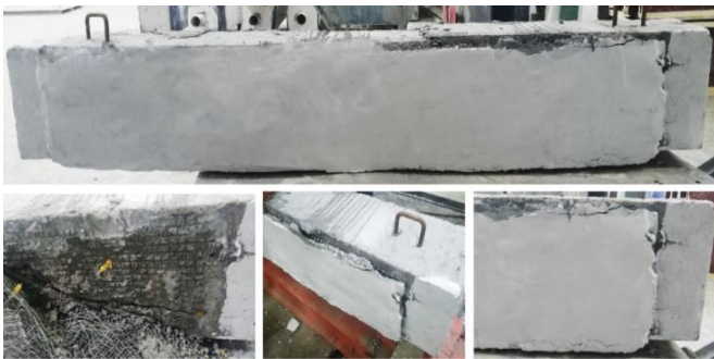
Fig. 13 The (S.-J. + Ferrocement) beam after the failure.
