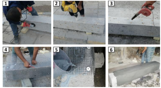
Fig. 6 The steps involved in the strengthening of the beam (S.-J. + Ferrocement).
