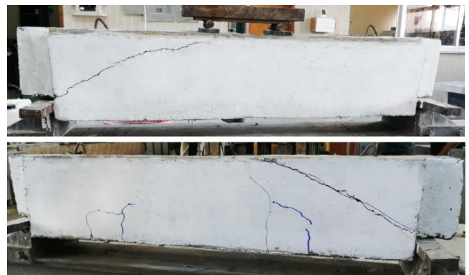
Fig. 11 The (S.-J. + Steel Fiber) beam after the failure.
