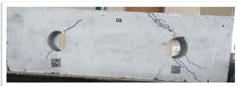
Figure 11. Shear cracks pattern of D8
