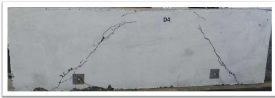
Figure 7. Shear cracks pattern of D4
