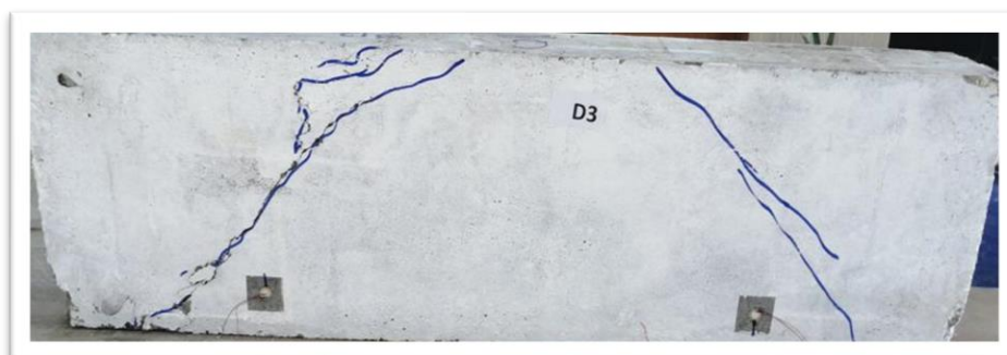
Figure 6. Shear cracks pattern of D3
