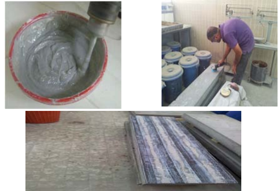
Fig. (3): Preparing and application of CFRP strips.
