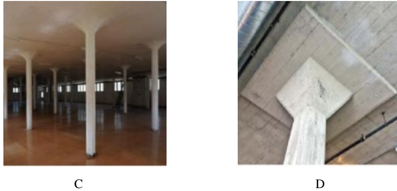
Figure (1): Types of flat slabs ( https://www.slideshare.net/satishhn/civil-structural-engineering-flat-slab-design )
