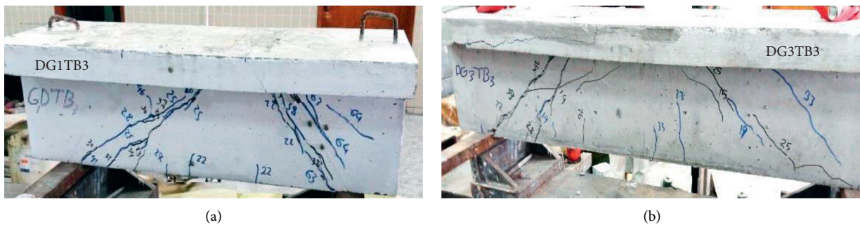
FIGURE 10: Crack pattern for directly loaded beam (DGTB).
