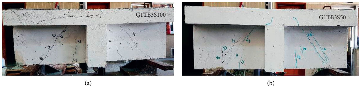
FIGURE 9: Crack pattern for indirectly loaded beams with shear reinforcement.
