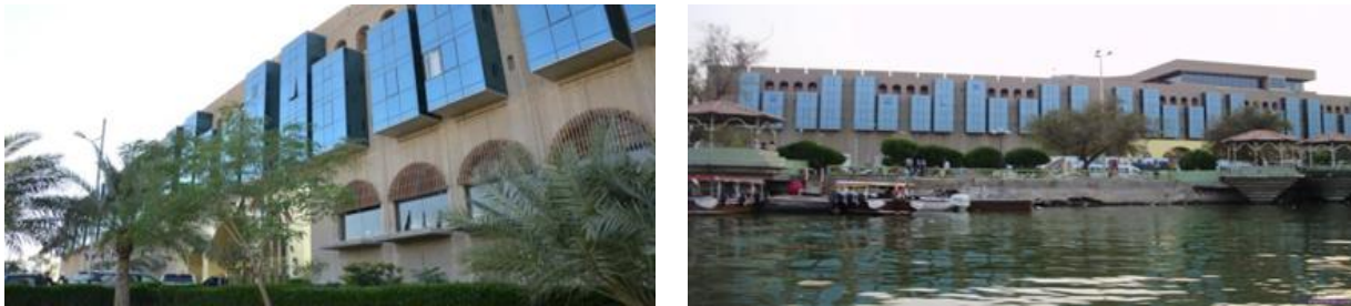
Figure 12. Sheraton Hotel after the reconstruction and replacement of the wooden Schnachil glass panels with packaging
