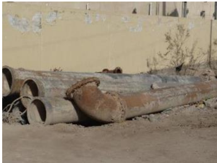
Rusted pipes in Al Chebayish
