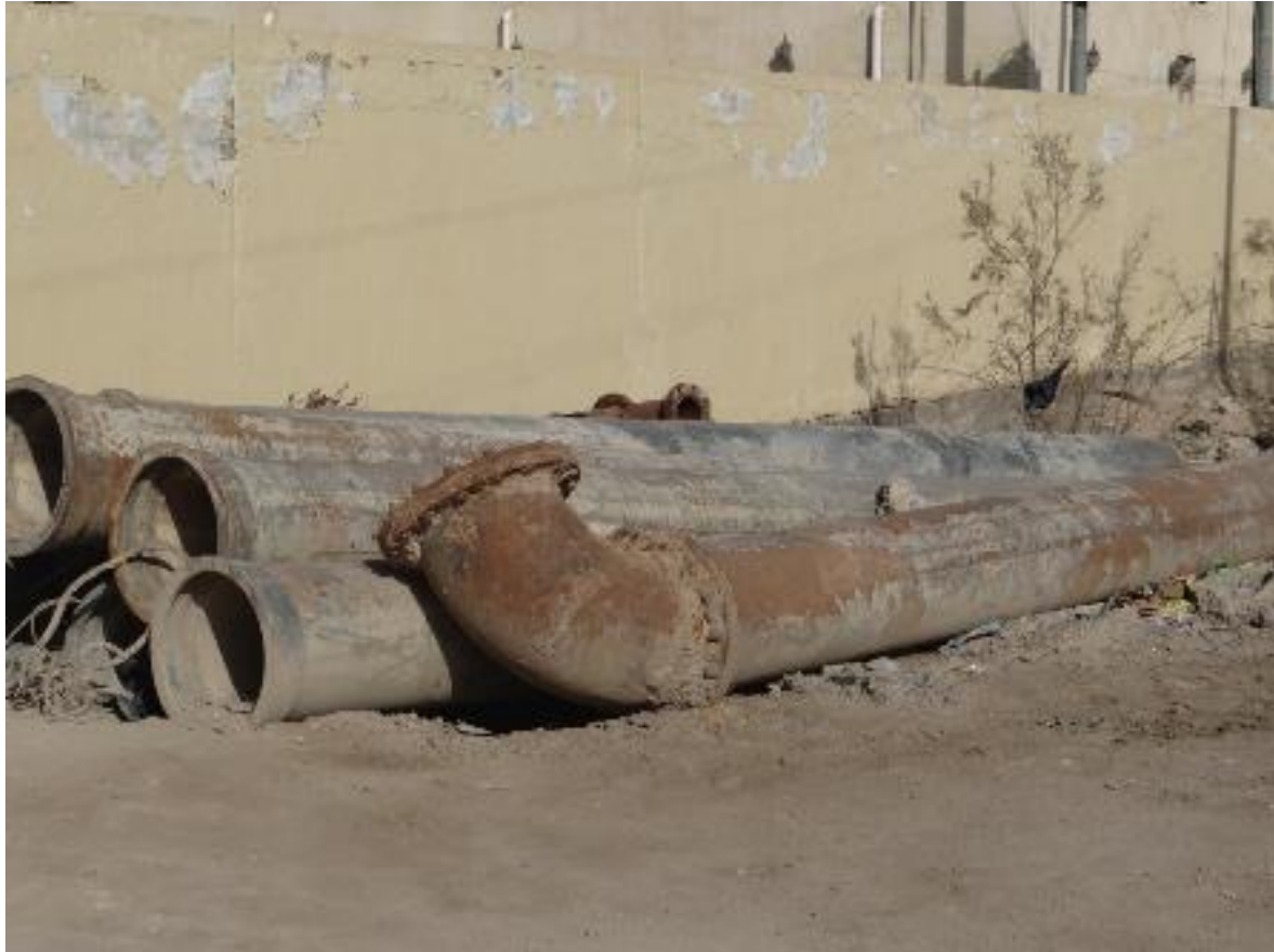
Rusted sanitation pipes in Al Chebayish town, Dhi-Qar governorate
