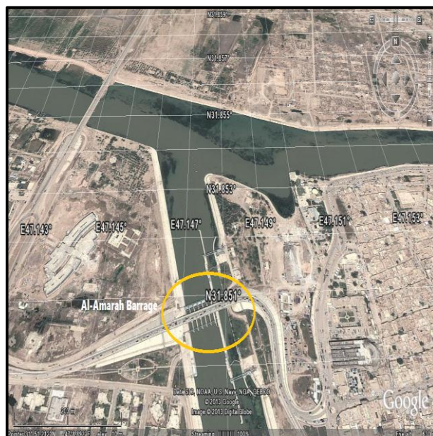
Figure 2. Location of Al-Amarah Barrage [18]
