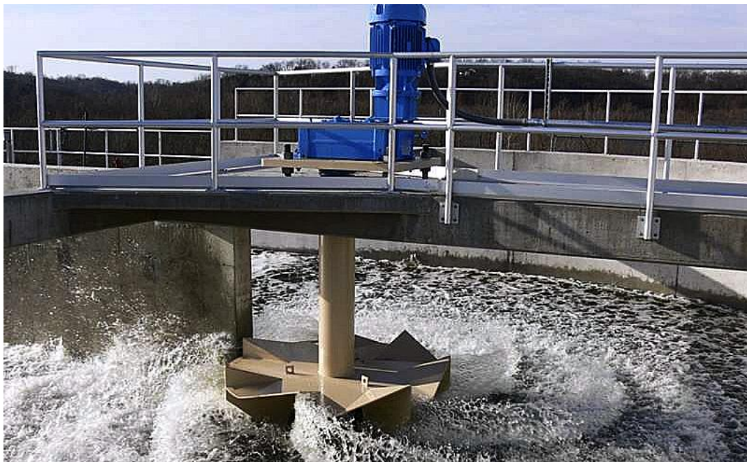
Fig.(4-11) Mechanical surface aerator
