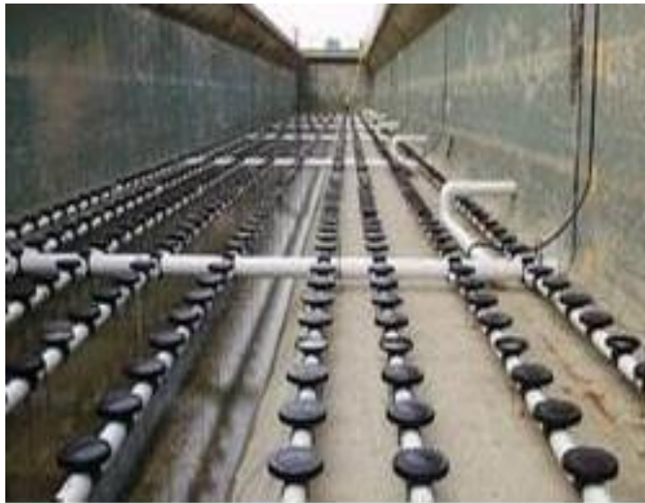
Fig.(4-10) Diffused aeration system
