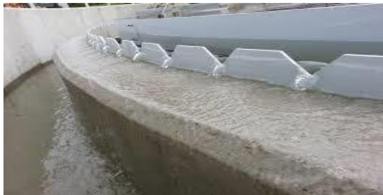
Fig.18 V-notches outlet weir
